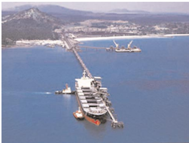
North Pulau Laut Coal Terminal
