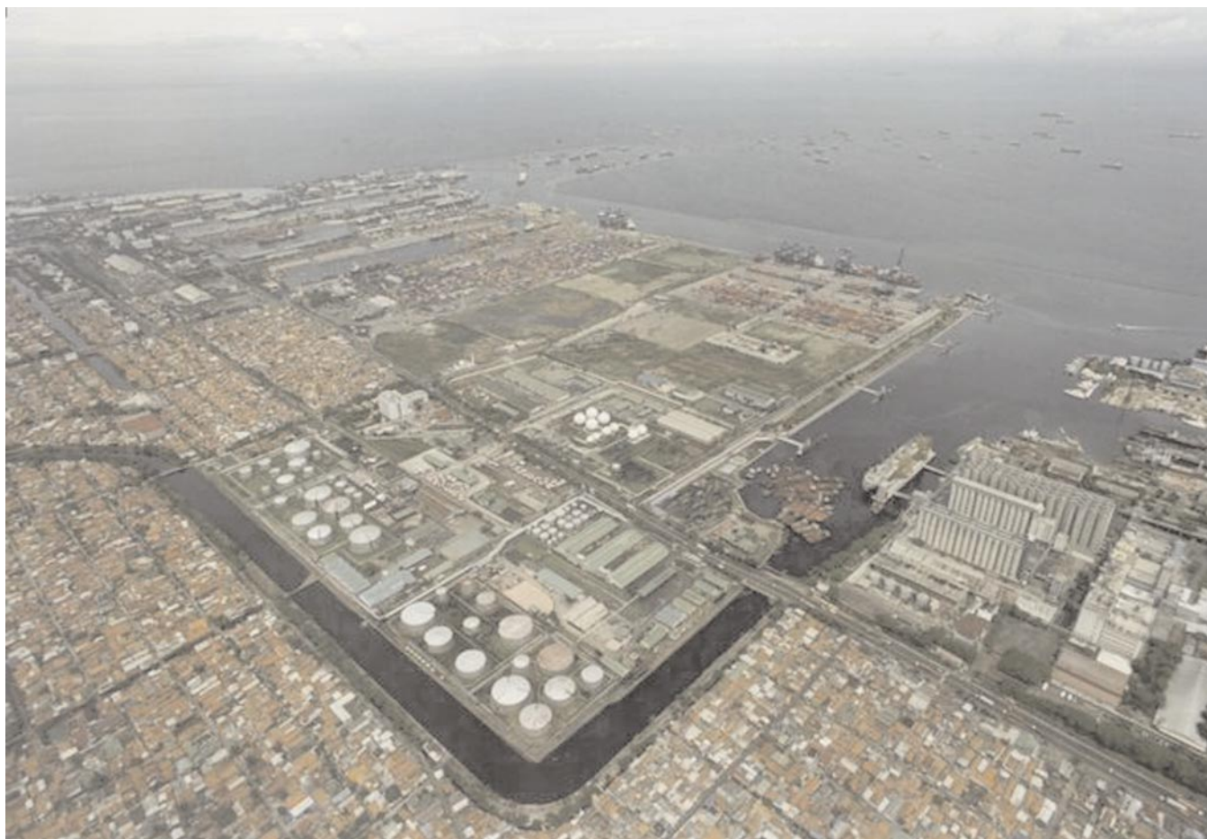
Aerial Image of Tanjungpriok
